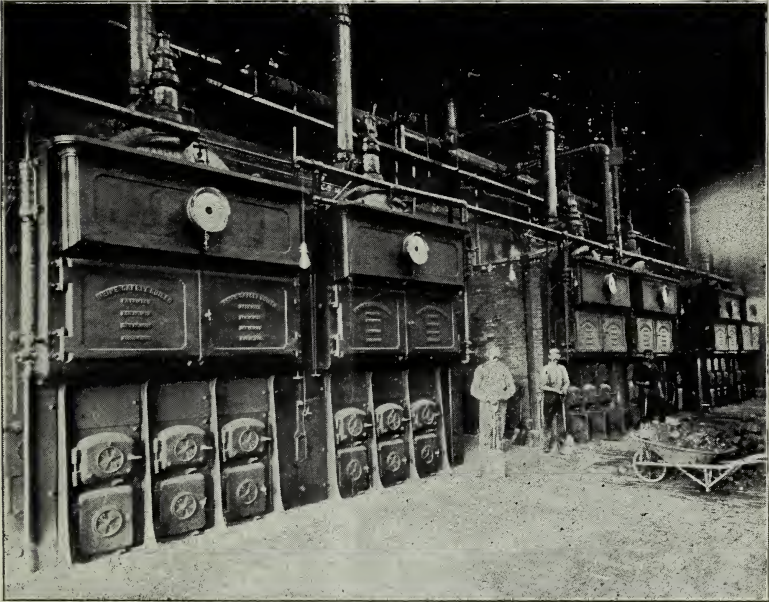
View of Boiler Room, Pumping Station of the Peoria Water Co.
